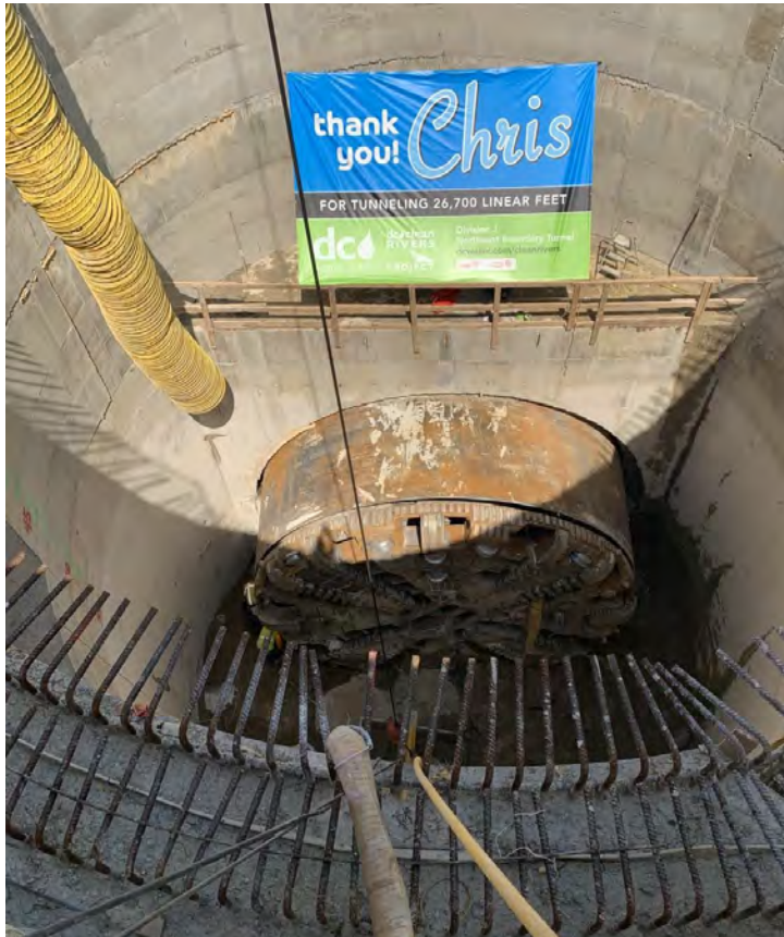
Northeast Boundary Tunnel Hole Through at 6 th and R St NW
