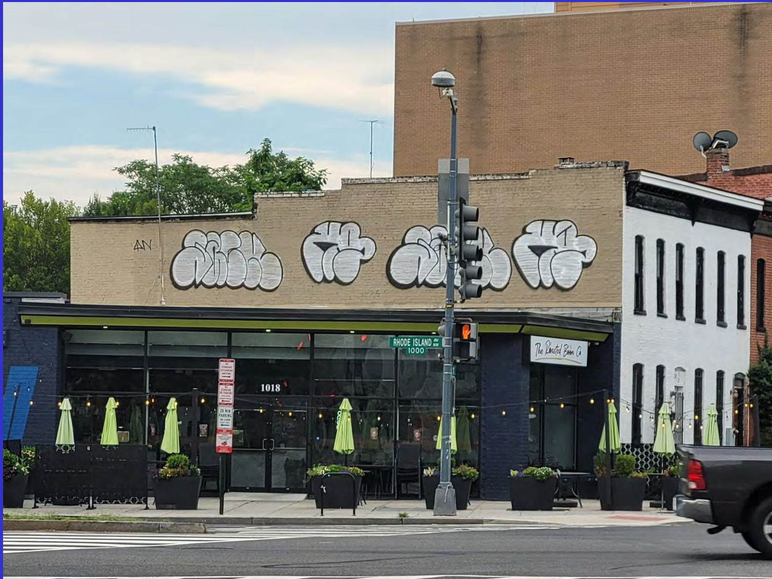
1521 11 th STREET, NW: CURRENT APPEARANCE
