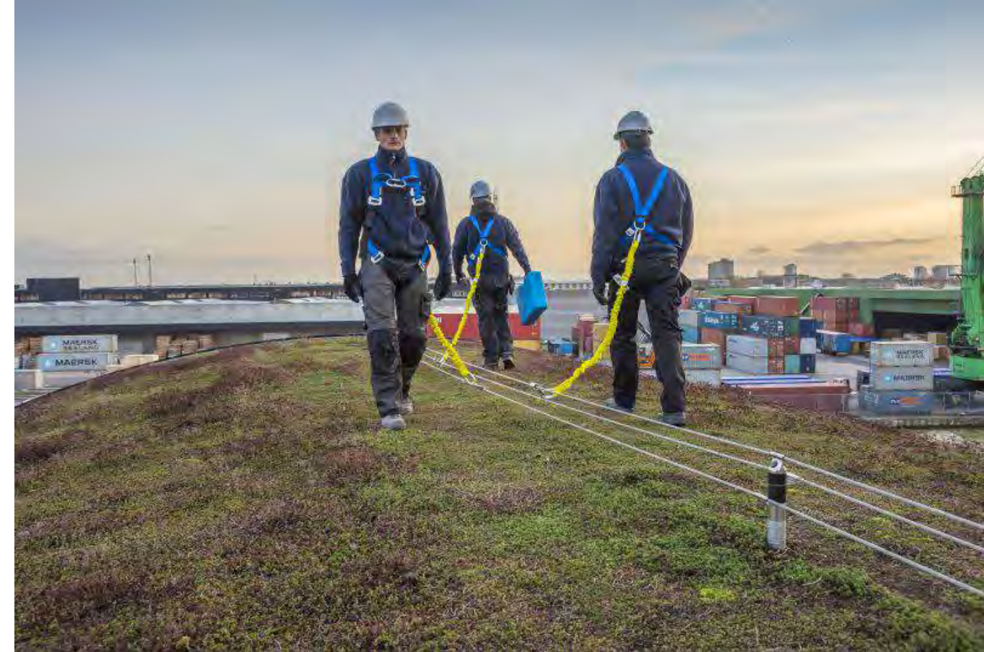
EXAMPLE OF SAFETY TIE BACKS IN USE
