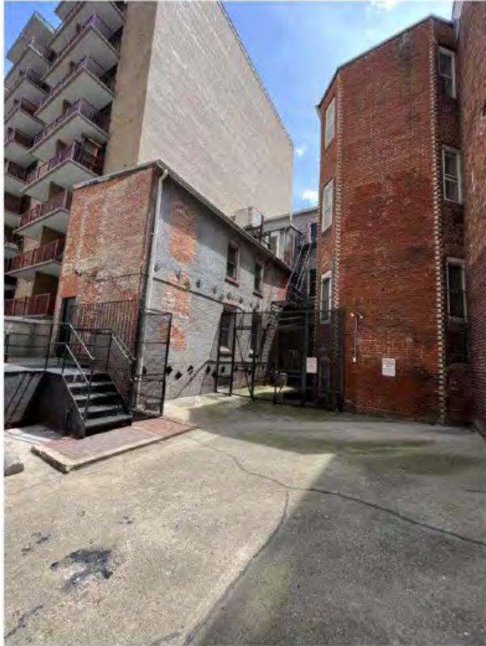
① EXISTING REAR VIEW ROAD: N/A
