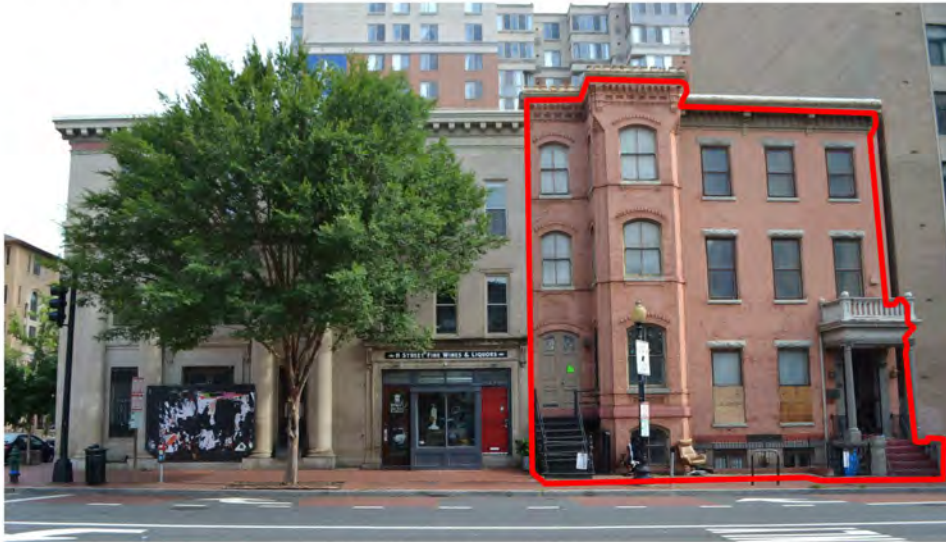
Existing Front Façades of 471, 473, 475 & 477 H Street NW
