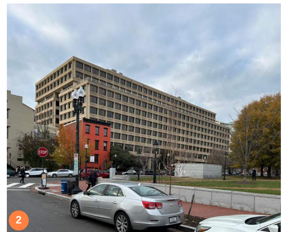
EXISTING BUILDING PHOTOS
